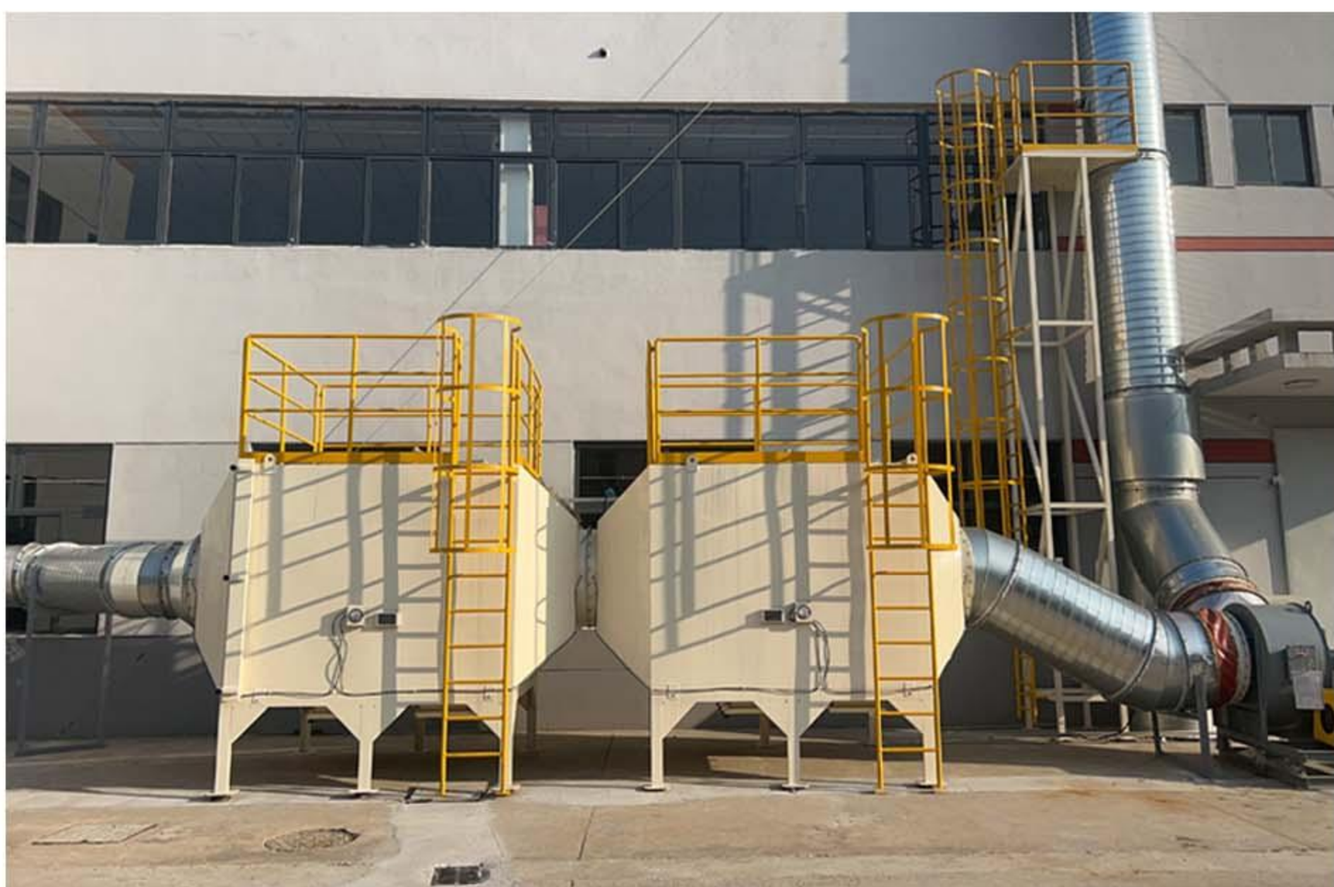
Power Industry in Suzhou VOCs Secondary Adsorption Purification for Injection Molding
