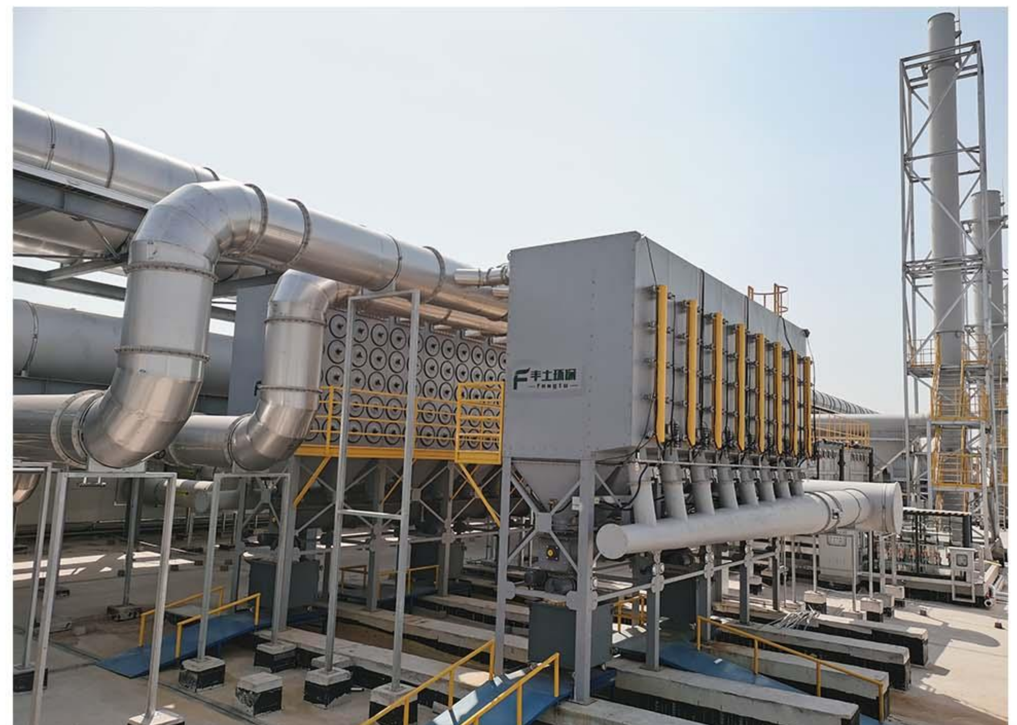
Optoelectronics Industry Dust Collection System - Zhengzhou
