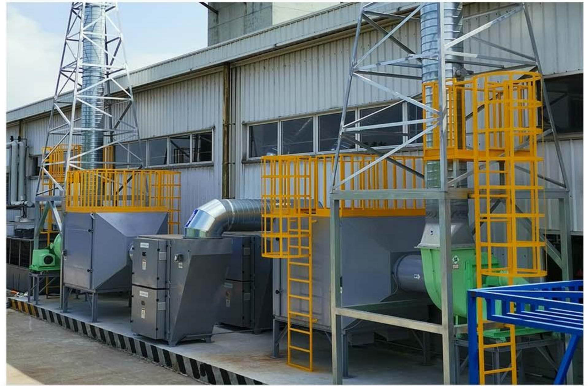
Japanese Glass Industry Enterprise in Suzhou VOCs Secondary Adsorption Purification System
