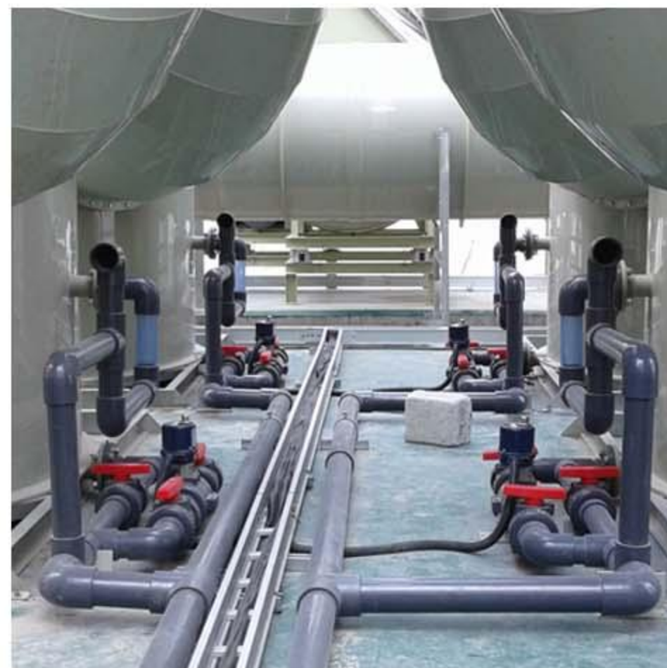
Overflow Port and Inlet Positioned at 180°
