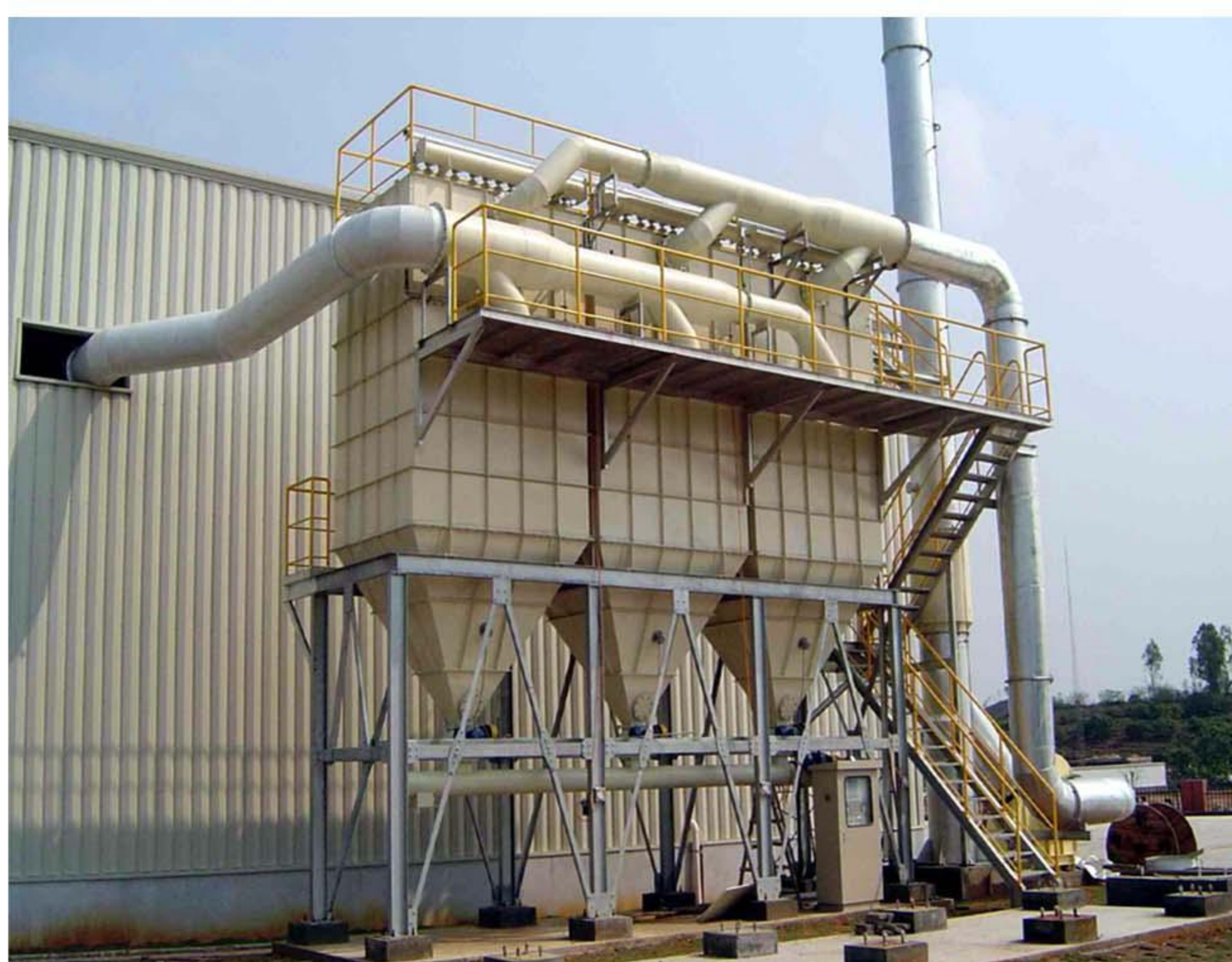
Dust Collection System for Automotive Parts Industry - Guangzhou
