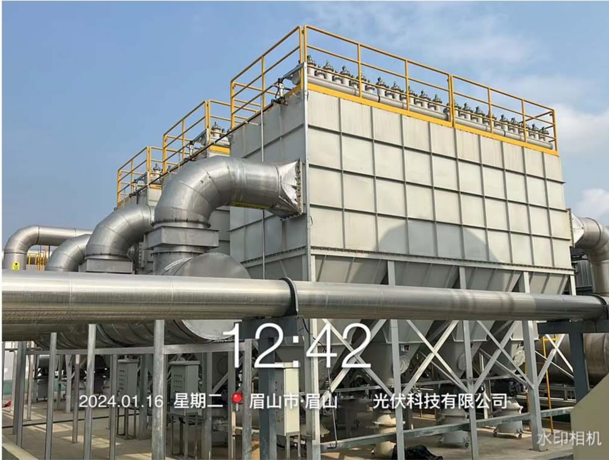
Topcon Process Dust Collection System for Photovoltaic Industry - Meishan, Sichuan
