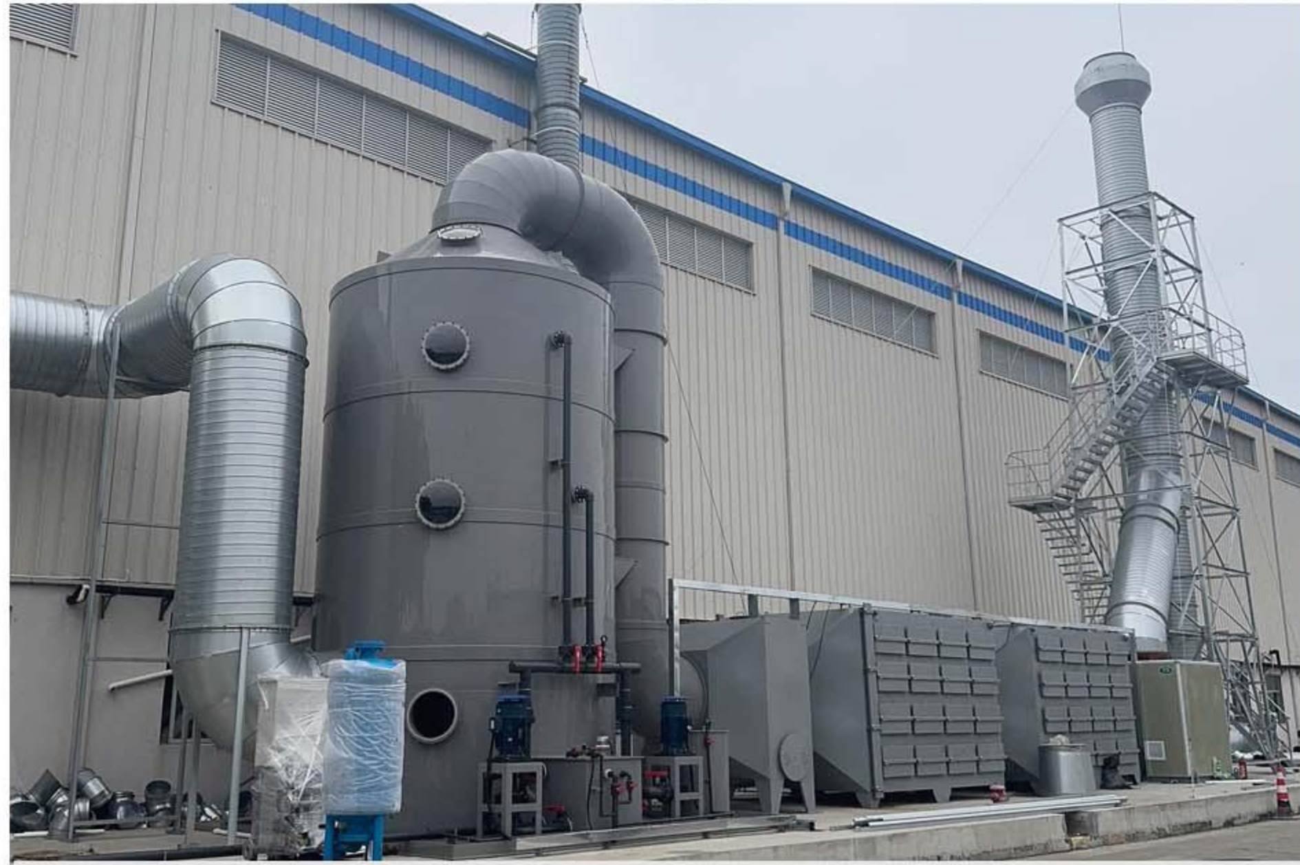
BYD Injection Molding Workshop in Shanwei VOC Exhaust Treatment, 58,000 CMH
